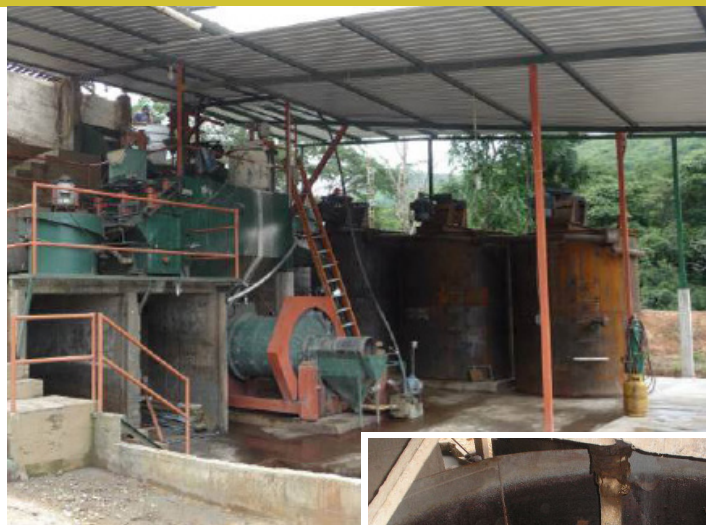
(Above) The demonstration plant in Portovelo, Ecuador for education and training of artisanal miners. (Right) A grinding mill with rotating cement wheels common in Portovelo. Photos: Jane Dennison
